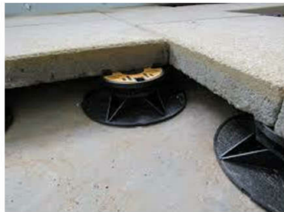
EXAMPLE OF POD AND PAVER SYSTEM
